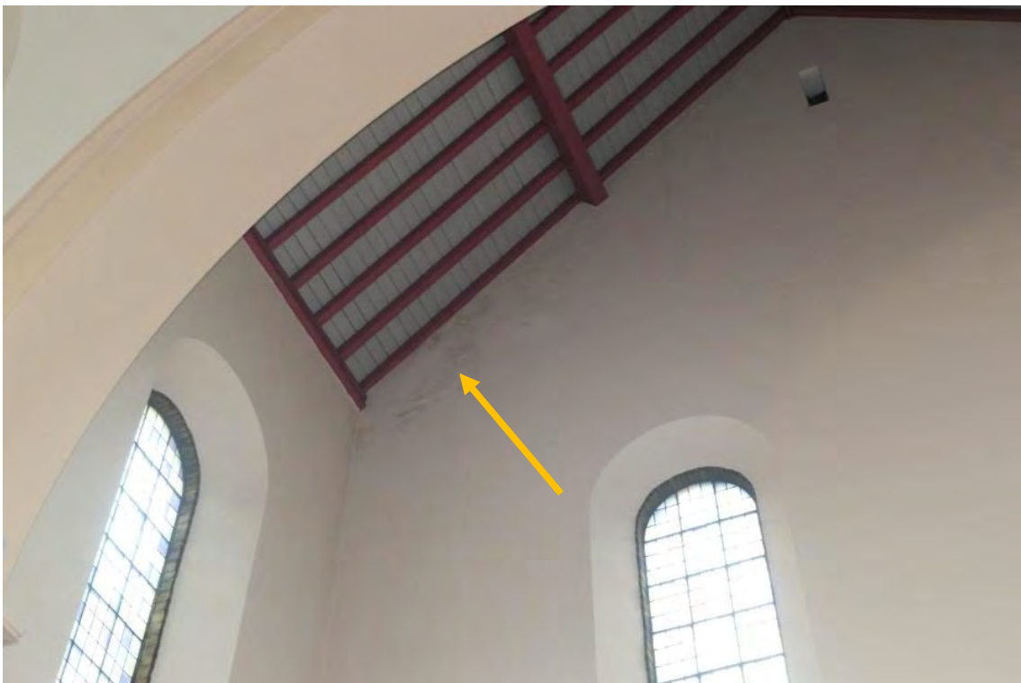
Photo 14 (Below): Overview of damp staining to the top left side of the gable end to the west transept.
