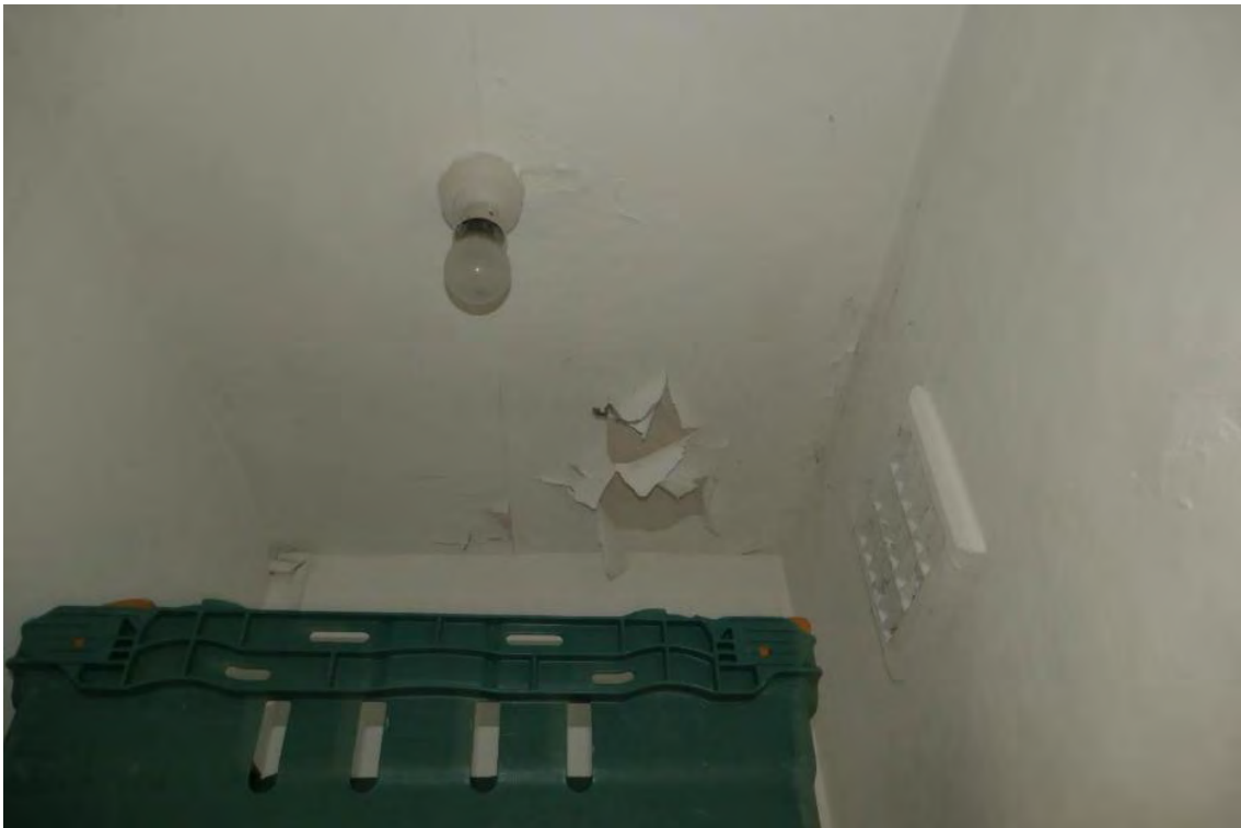
Photo40 (Below): Overview of peeling paint within the utility cupboard of 3 Hamilton Road.
