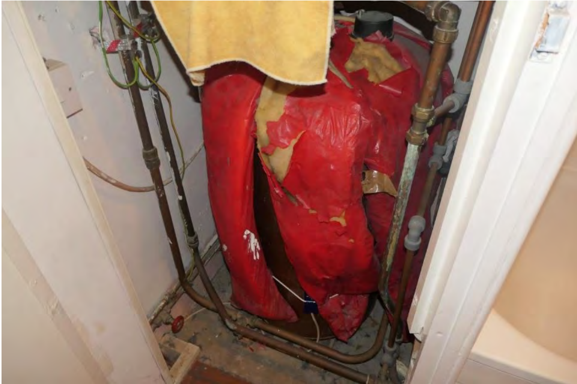
Photo40 (Below): Overview of peeling paint within the utility cupboard of 3 Hamilton Road.
