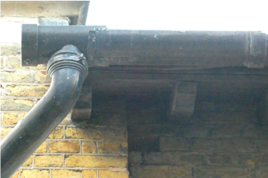
Photo 10 (Below): Overview of the rainwater goods to the east elevation of the church showing poor guttering detail to the church. There is a leak in this location that has caused staining to the roof tiles below.
