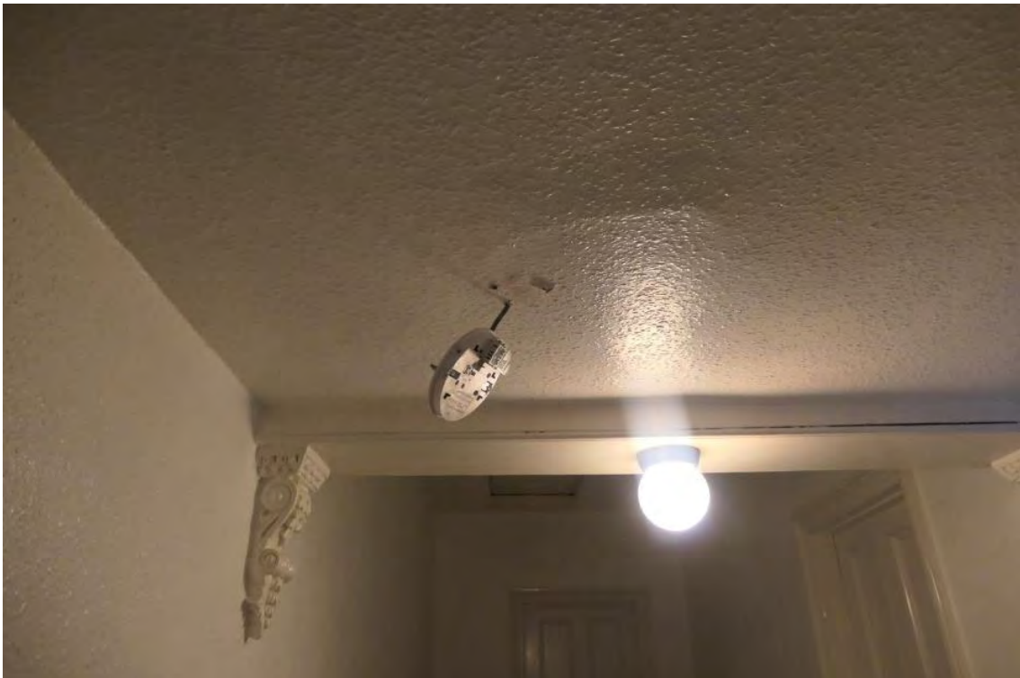
Photo 28 (Below): Overview of a loose smoke alarm detector to the first floor within 1 Hamilton Road. The first floor is currently not used and requires refurbishment.
