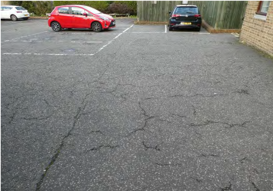
Photo 12 (Below): Overview of surface cracking to the car park surface. Renewal of the car park and access road surface will be required in the medium term as the cracks widen.
