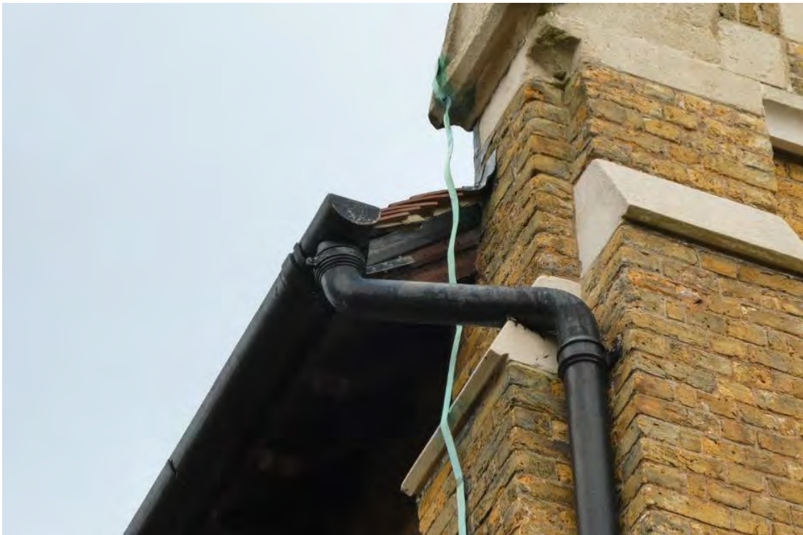
Photo 6 (Below): General overview of loose lightning conductor strip to the west elevation of the church.
