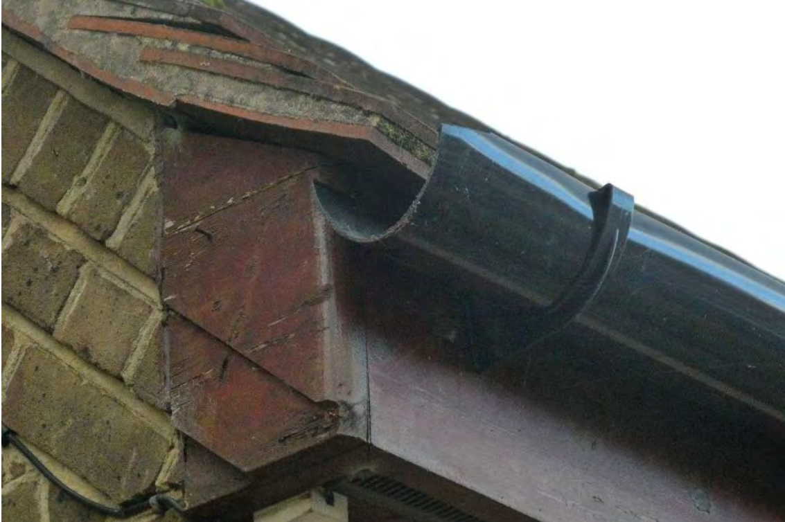
Photo 10 (Below): Overview of the rainwater goods to the east elevation of the church showing poor guttering detail to the church. There is a leak in this location that has caused staining to the roof tiles below.
